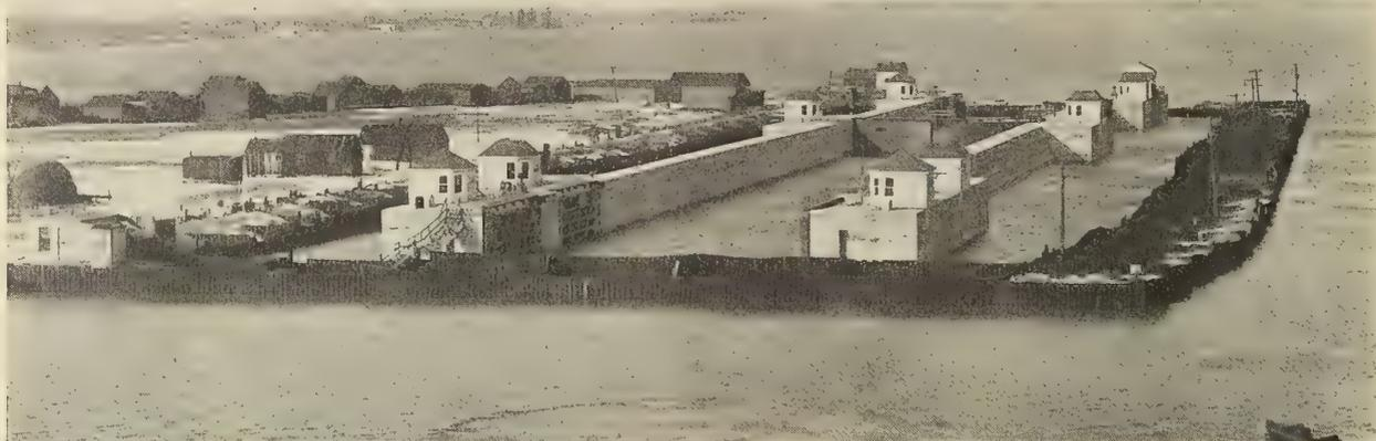
Completed lock ready for withdrawal of piling and at the time the United States Government was testing the tightness of lock gates preparatory to acceptance.
